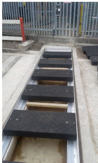
Fibrelite covers and frames were custom made to fit existing apertures, minimising installation time / upheaval to site
