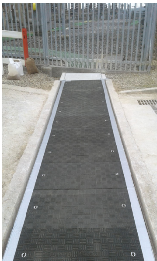
Fibrelite covers and frames were custom made to fit existing apertures, minimising installation time / upheaval to site
