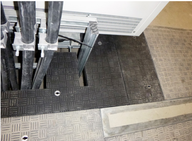
Custom Fibrelite trench access covers designed with cut-outs to accommodate piping and cabling
