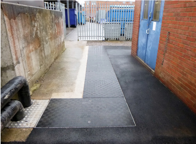
Bespoke Fibrelite covers provide safe replacement for previously installed concrete covers
