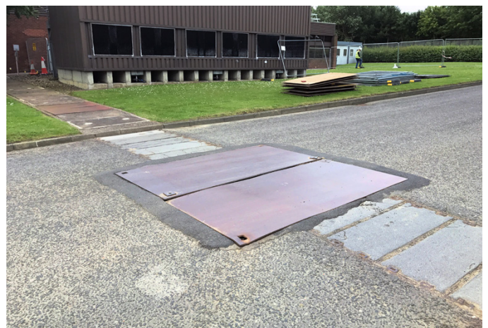
Previously installed failing concrete and metal covers
