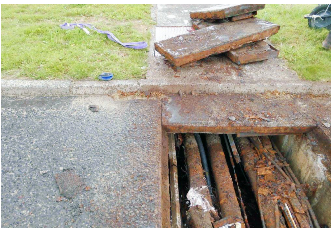
Previously installed heavily corroded access covers
