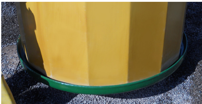
Fibrelite's 42" E85 compatible tank sumps being installed on double wall steel tanks
