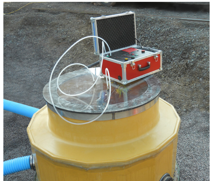
Vacuum testing to ensure a watertight installation
