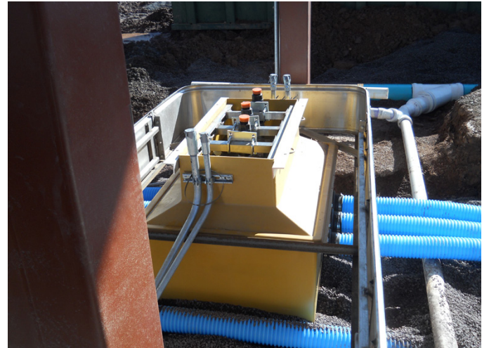
Fibrelite's E85 compatible Encore 500 dispenser sumps
