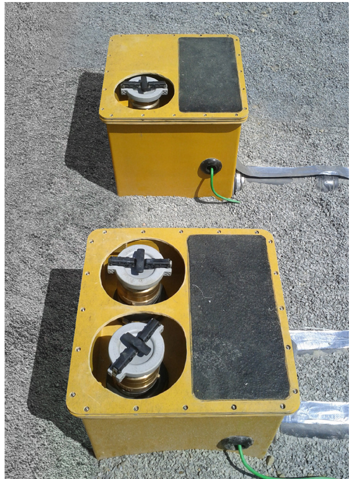
Secondarily contained Fibrelite remote fill sumps with anti-slip step down platforms
