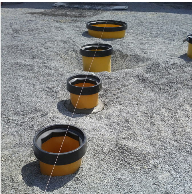
Fibrelite's manual dip and interstitial monitoring sumps being installed
