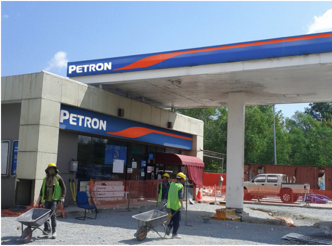
Site under construction
