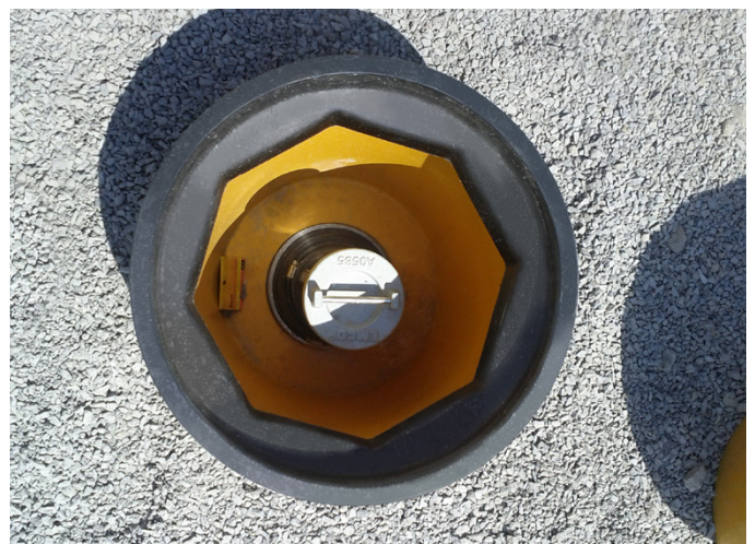
Fibrelite's watertight vacuum tested manual dip sump
