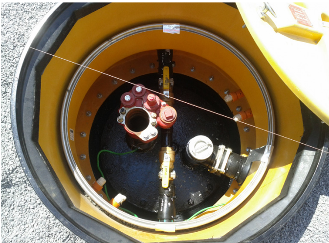
Fibrelite's 1.2m 16 sided turbine sumps being installed
