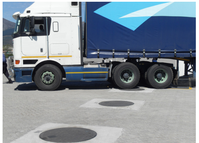
Fibrelite cover installed in truck lane
