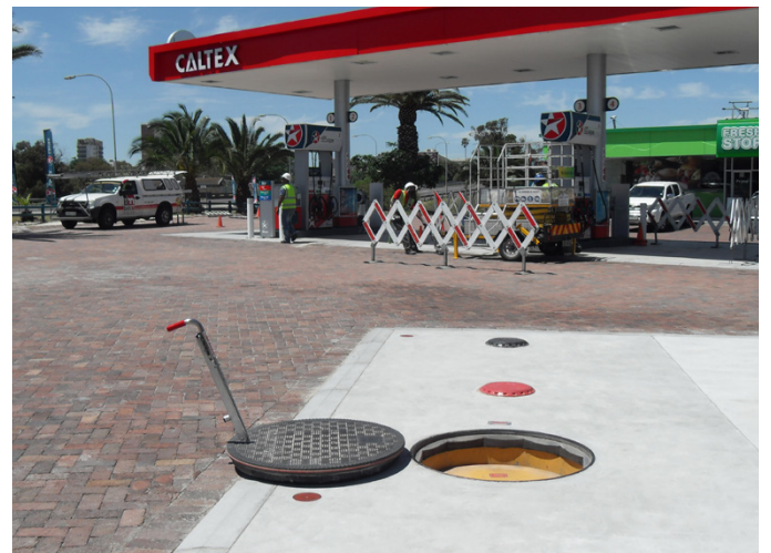
Watertight Fibrelite covers and tank sumps
