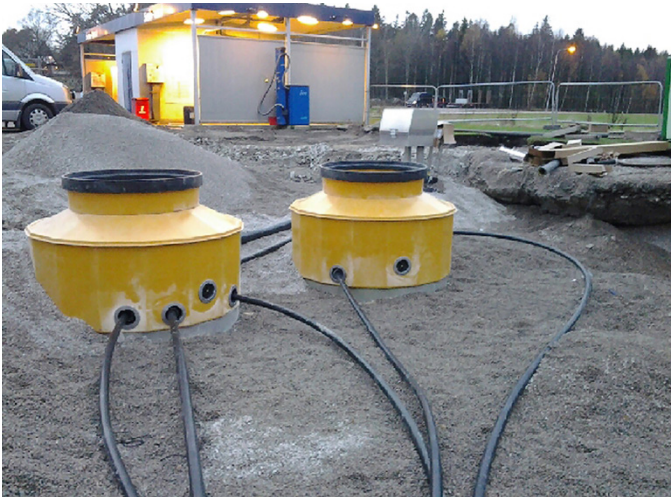
Newly designed 1.7m (S17) diameter tank sumps being installed in Norway
