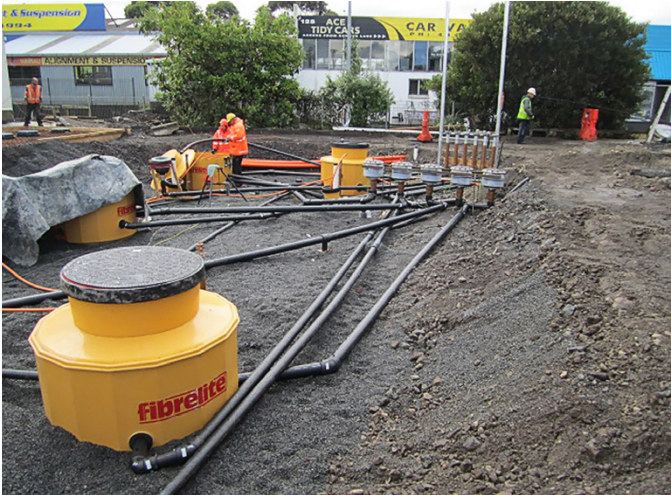
Fibrelite sumps are vacuum testable ensure watertightness
