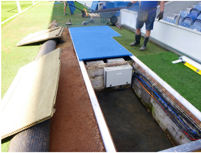
Fibrelite installed a range of lightweight covers which can be removed and replaced by two people using the ergonomically designed FL7 lifting handles
