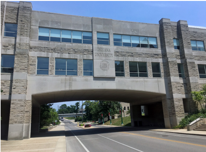
Indiana University required steam rated manhole covers
