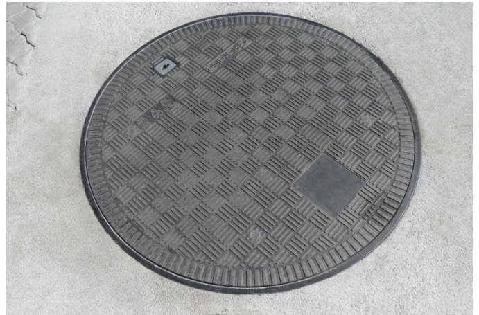
Fibrelite installed (FL 90) with a 40-tonne load rating
