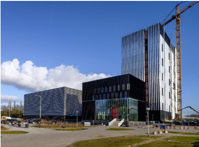
Fibrelite trench covers protect fibre optic cabling at emergency vehicle access point (image used for illustration purposes as actual data centre cannot be shown)
