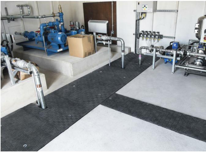
Two different load rated covers were used for the installations, B125 and D4.00
