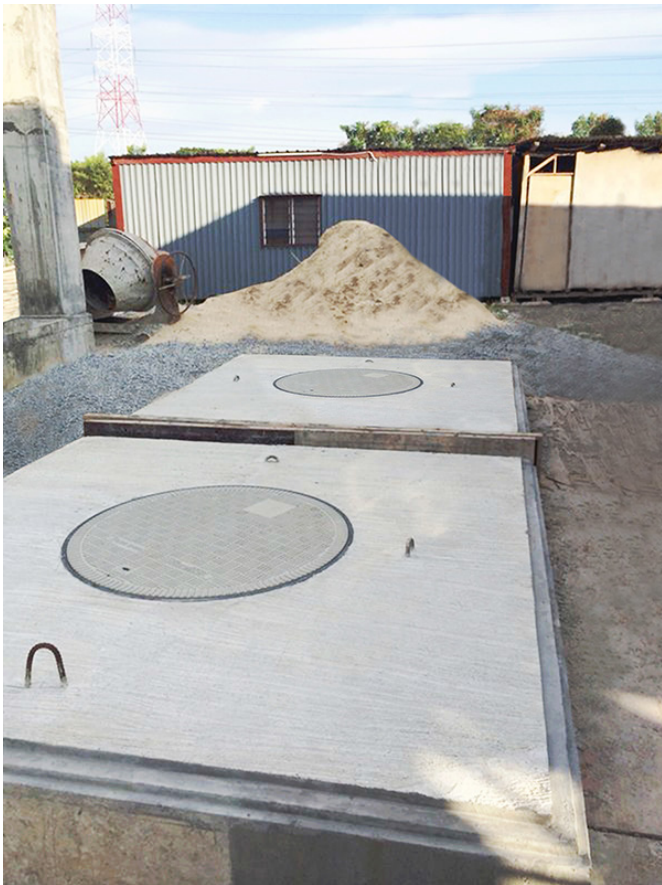
Plinths ready for installation
