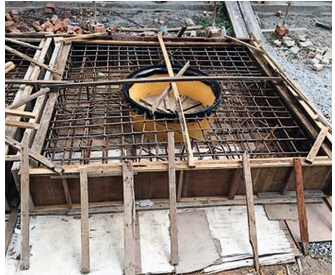
Prefabricating concrete plinth with Fibrelite FL90 frame
