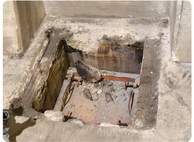
Old access frames can easily be removed and replaced with Fibrelite frames
