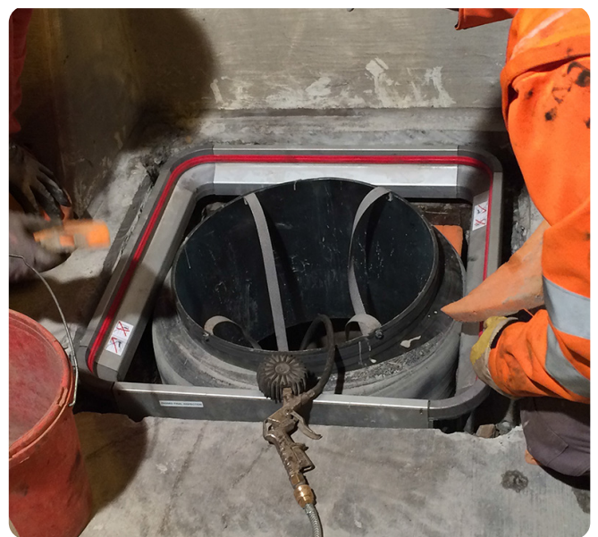
Fibrelite covers will not rust and degrade like metal and concrete covers
