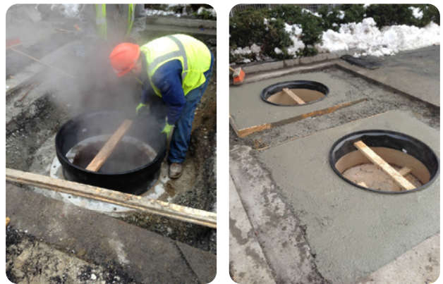
Fibrelite installations are simple – a fiberglass skirt can be used as a preform and to set the frame at grade
