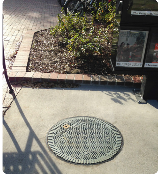
Lightweight composite steam cover - Product code F65
