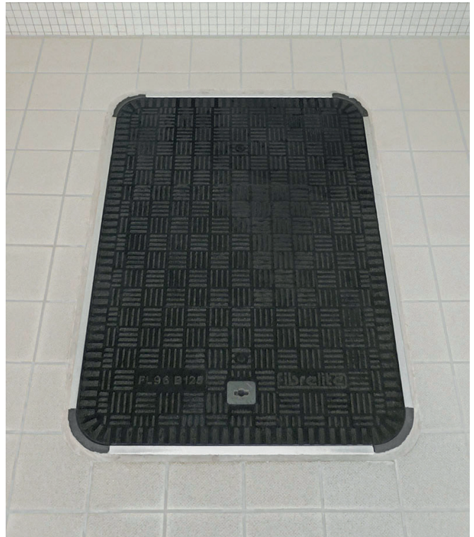
Fibrelite's FL96 watertight manhole cover installed
