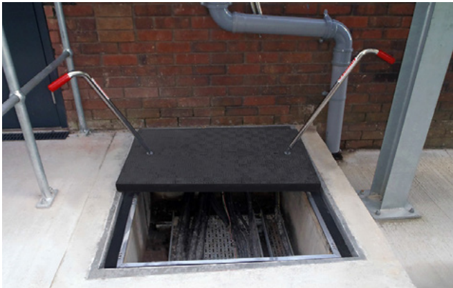
Sealed Fibrelite covers prevent water ingress
