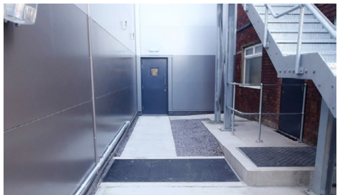
Retrofitted sealed Fibrelite covers installed
