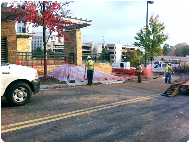
Road before concrete vault and trench cover installed
