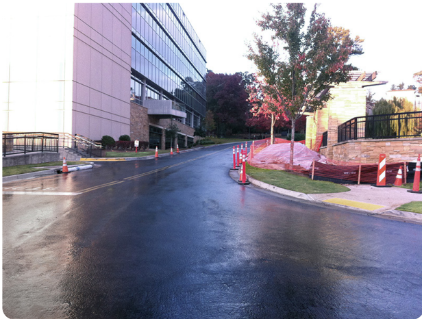
Pre-install location for the Fibrelite covers
