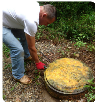
Heavy cast iron covers pose a significant threat of back & shoulder injuries along with the risk of trapped extremities
