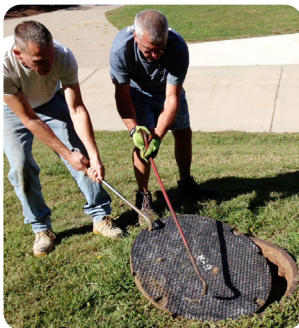
Heavy cast iron covers pose a significant threat of back & shoulder injuries along with the risk of trapped extremities
