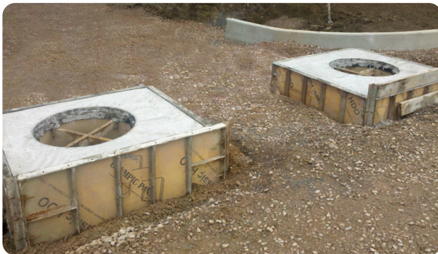
Pre-cast Fibrelite frames
