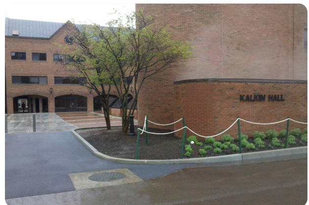
Fibrelite composite FRP cover installed in frame
