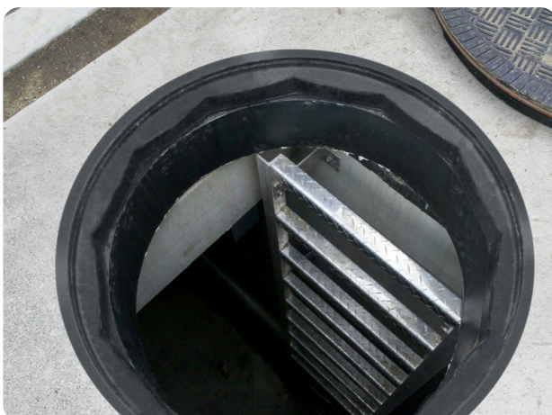
View from over the manhole
