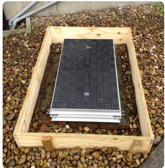
Single FM45 ready for new concrete to be poured
