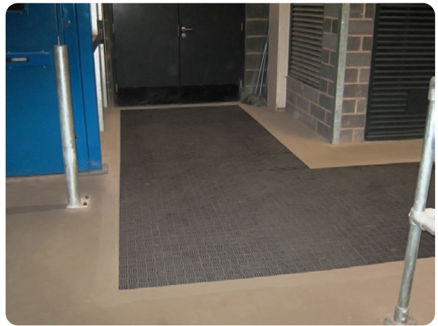
Fibrelite's trench panels can be used to cover large areas and corners
