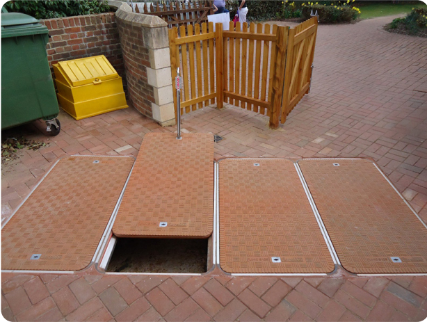
Newly installed Fibrelite flat sealed FL140 composite covers
