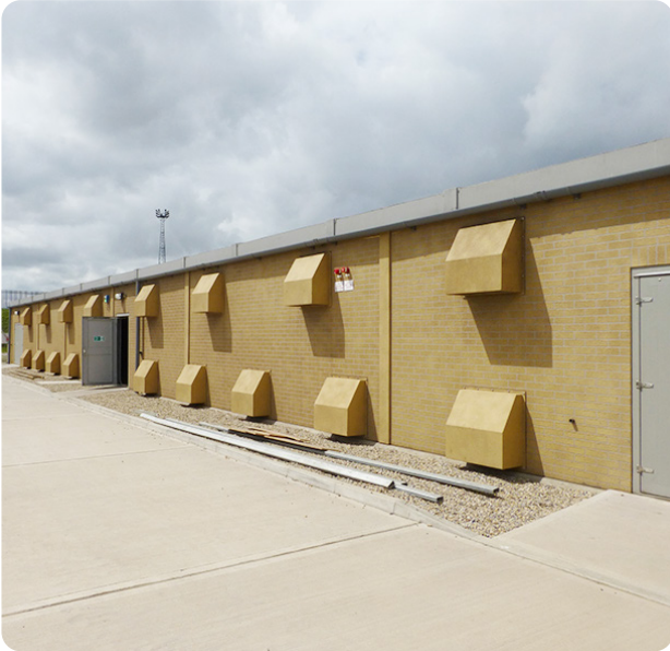
UK Gas Valve Plant
