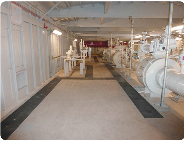
Special notched panels have been fitted around valves and pipework
