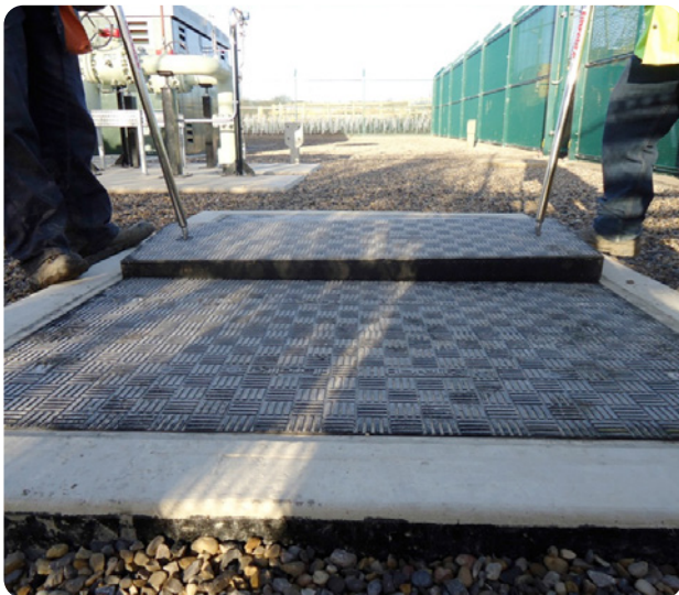
Trench panel being lifted easily using Fibrelite's FL7A lifting aid
