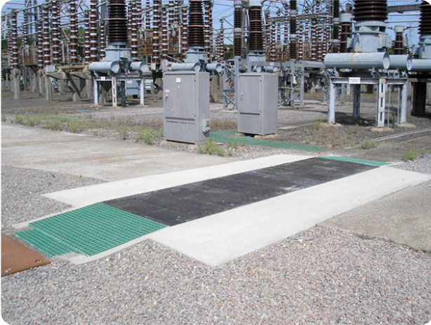
The Fibrelite D400 tonne load rated lightweight trench covers
