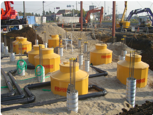
Fibrelite's 1.4m 16 sided tank sumps being installed
