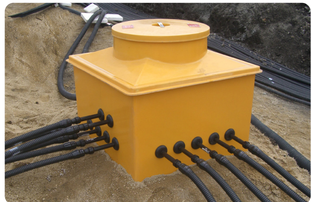
Fibrelite's electrical conduit drawpit being installed
