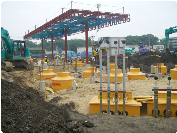
Site under construction
