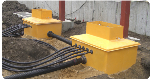
Fibrelite's Tokico AB26L dispenser sumps
