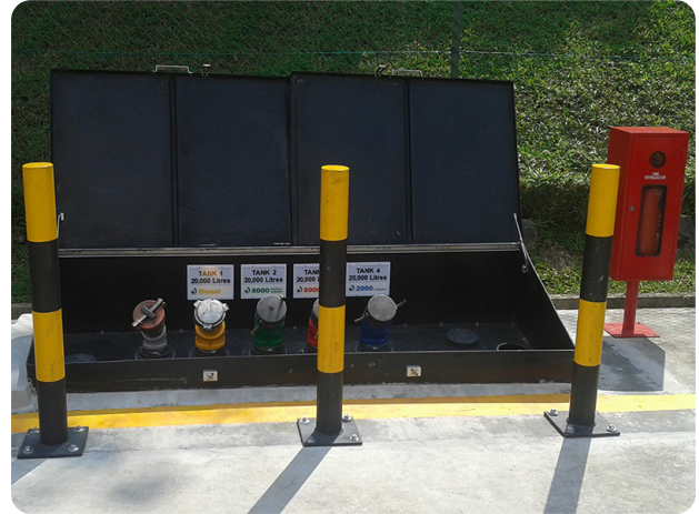
Fibrelite tank sumps being installed
