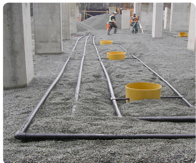
Network of pipes buried in the ground
