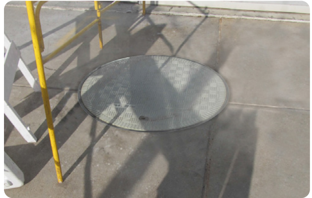
Fibrelite F95 composite cover installed in frame
