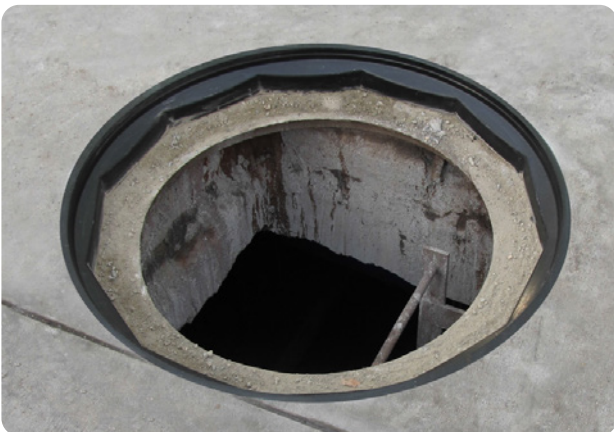
Fibrelite composite frame installed in sidewalk
