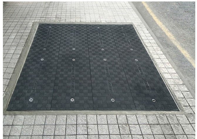
Lightweight GRP composite trench covers
